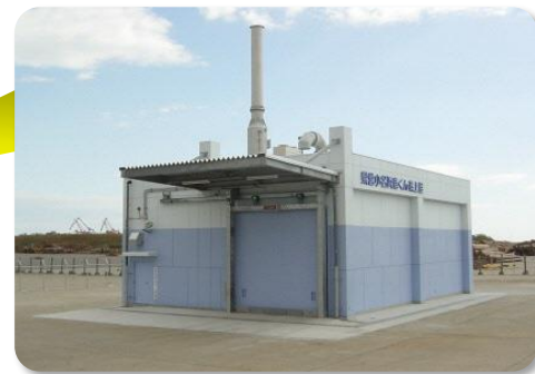
■小名浜港くん蒸上屋 (面積: 165.0㎡) Onahama Port Fumigation shed
